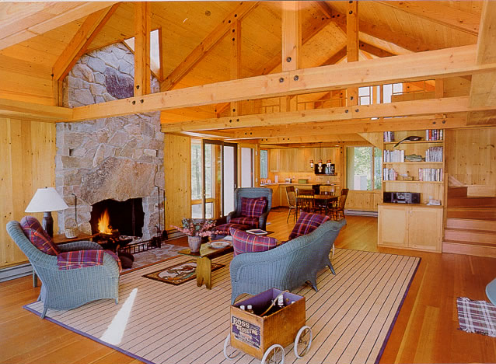
Modular rusticity. The living areas are unified beneath shop-built bents, spaced 6 ft. 8 in. o. c. to accommodate stock Andersen windows. A native-granite fireplace with a glazed chimney cricket up top occupies one module. The stair (right in photo) leads to a loft over the dining and kitchen areas.
