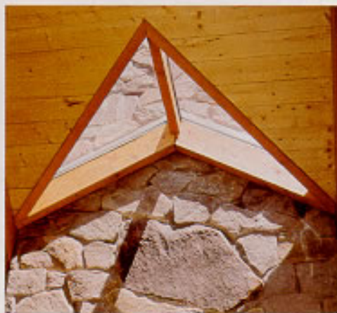
The glazed chimney cricket allows direct sunlight to wash down the face of the fireplace.
